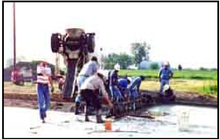
The concrete crew in action pouring 31st Street in Central City.
